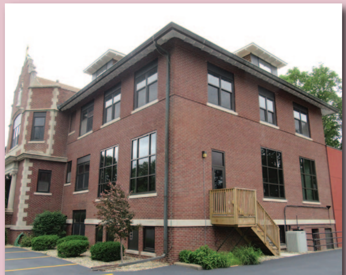
New windows and door for the Literacy Room, replacing the original stained glass windows and the original door that were all deteriorating.
