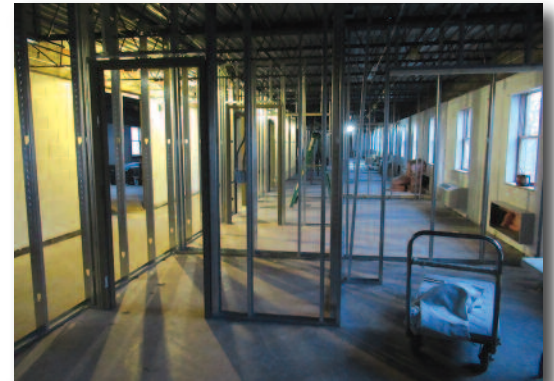
Framework for new bedrooms on 3rd floor.
